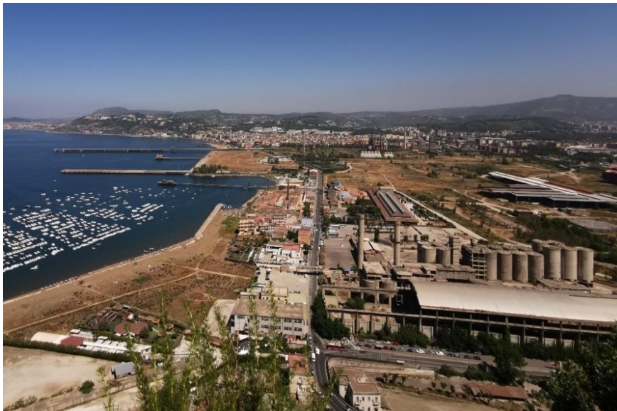
Figure 1. Ex-industrial area from Posillipo hill
