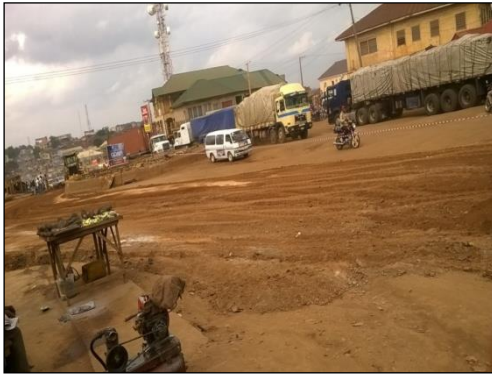
Figure 4. Road under construction
