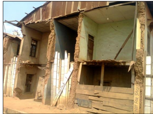
Figure 3. Demolished building for road expansion
