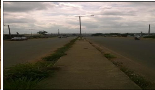
Figure 5. The dualized road with street light, drainage, and other facilities
