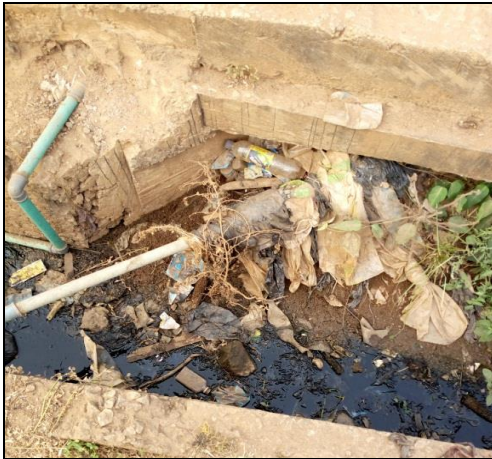
Figure 6. Storm Flow Obstruction by Utility Lines
