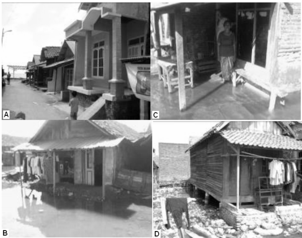
Figure 8. a) heightened housing foundation; b) inundated house; c) small dyke in front of the house; d) heightened housing type (rumah panggung)
